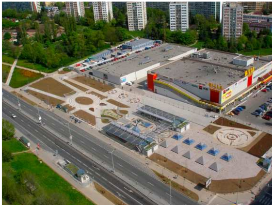
Fig. 2 Aerial view of the finished Prosek station
