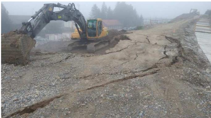
Figure 11. Slope adjustment without free cut
