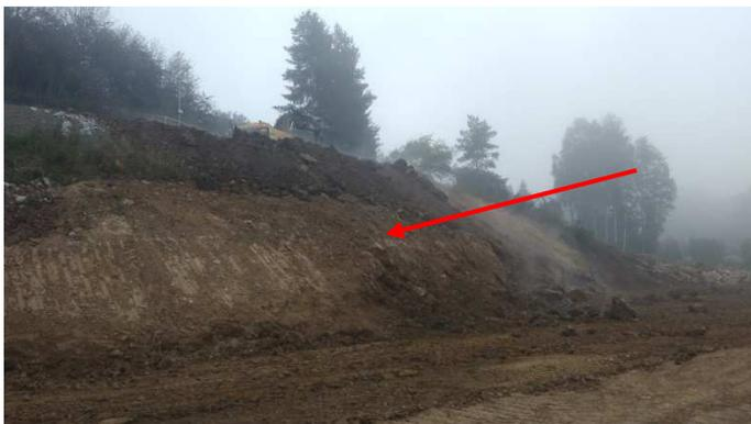
Figure 10. Slope adjustment without free cut
