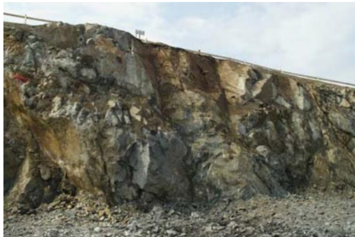
Figure 1: Western slope of the excavation pit, L. Marik photography
