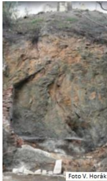
View on the rock slope – solve cross section
