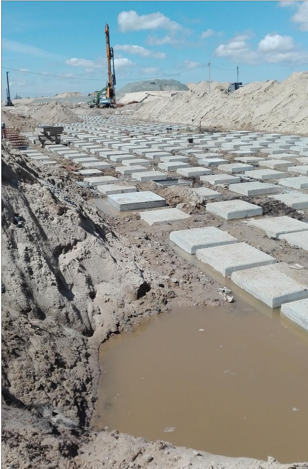
Fig. 5.5 Pile caps – reinforced slabs located on pile heads
