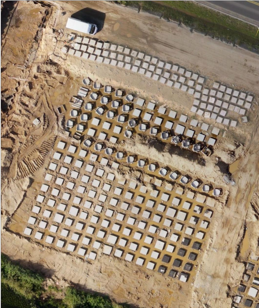
Fig. 5.4 Pile caps – reinforced slabs located on pile heads
