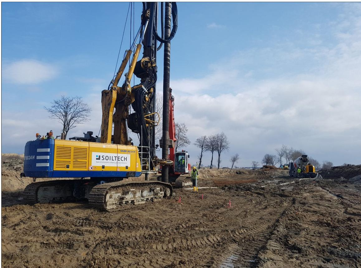
Fig. 5.1 Execution of displacement piles – rotary drilling rig BAUER BG 24 H
