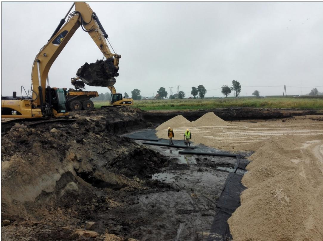
Fig. 1.1 Execution of soil replacement in km 29+375 S7
